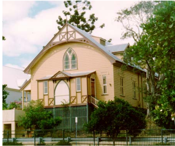
Former Petrie Terrace Baptist Church dating from 1895
