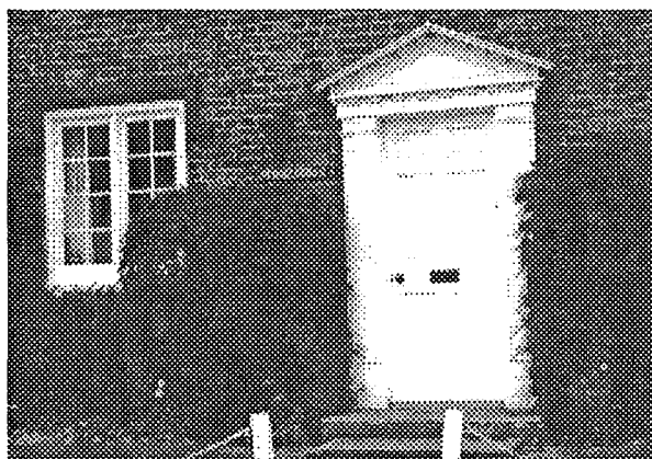
The Voller's residence at Bishop Burton, still in use as a private dwelling, and known as 'The Manse'. The main chapel building on the same site no longer exists (photo 1998)
